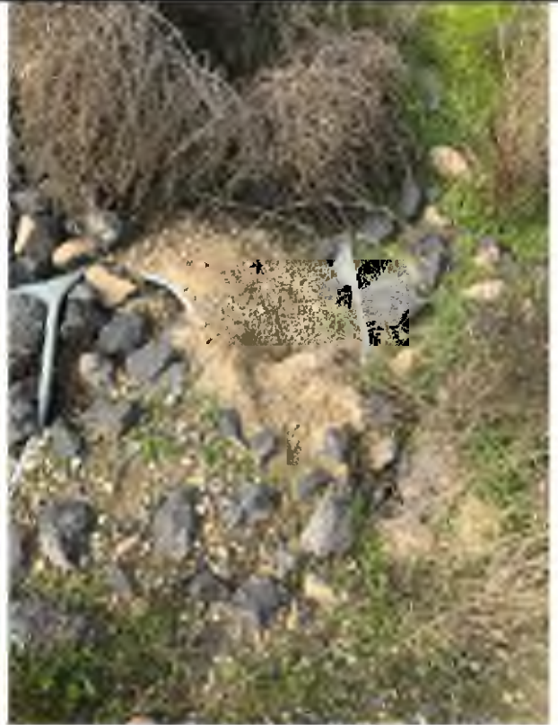
Filled slope drain now animal burrow
