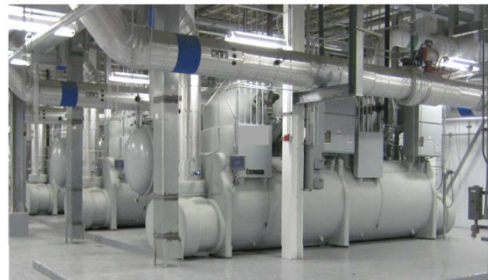
d) Large Capacity Water Cooled Chillers using Centrifugal Compressors
